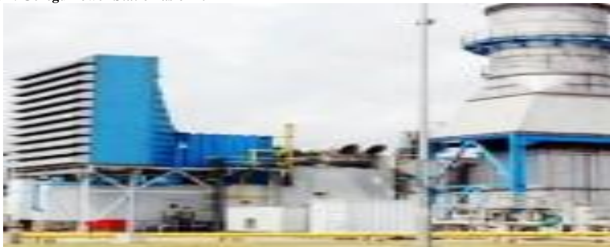
Figure 1: Geregu Power Station as of 2012
